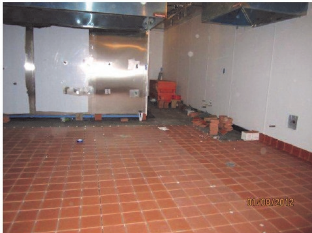
Kitchen, with floor tiles going in
