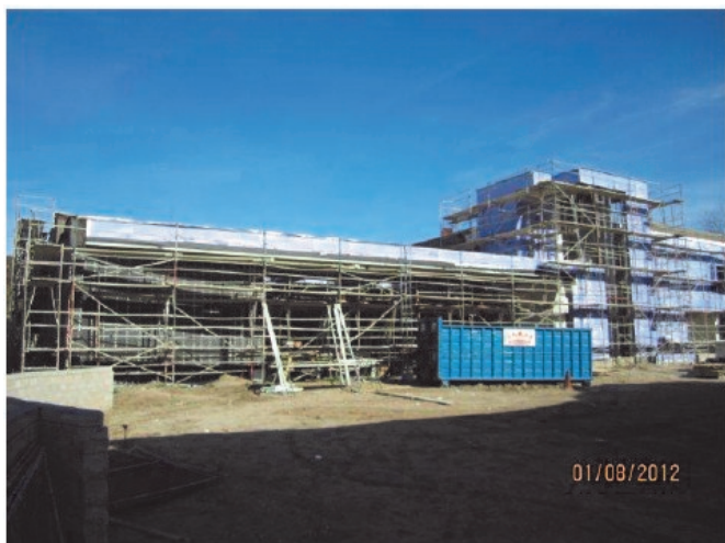
View from front of Church
