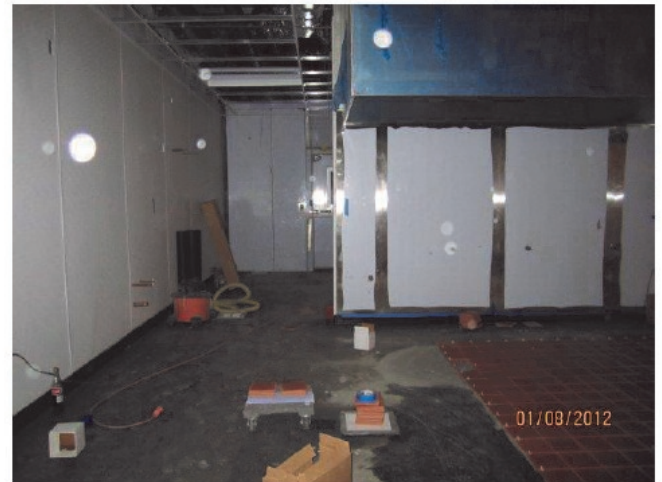
Kitchen, vent hood in foreground and walk-in refrigerator and freezer in back
